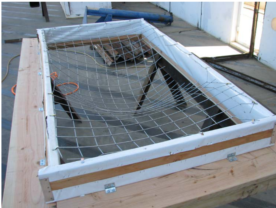
Photo No. 3 After removal of test weight
